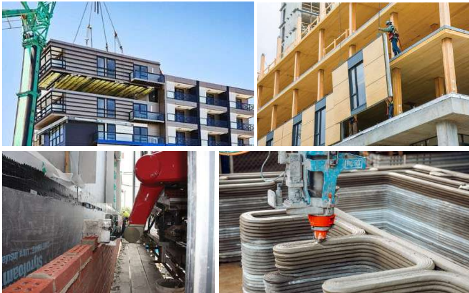
Fig. 6.3 : Advanced technologies : (Top Left) Modular construction, (Top Right) Mass timber construction, (Bottom Left) Robotic construction and (Bottom Right) 3D printing
